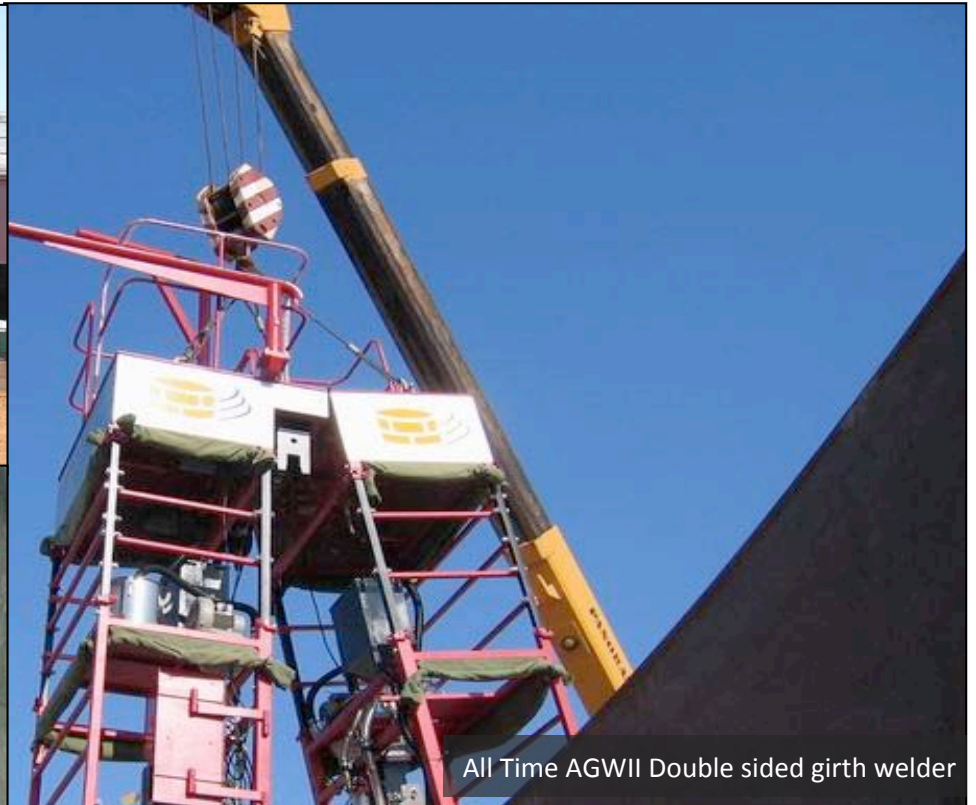
AGW-I/D welding "Jack Up" tanks
