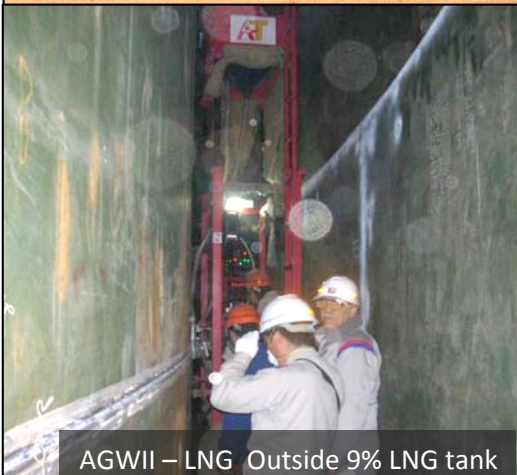
AGW-I/D welding "Jack Up" tanks
